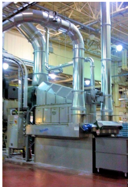
Above: Stainless 60 hp. HydroAIR, Double-Sided unit rated at 16,000 CFM at 12" External with all options and Turnkey Installation
