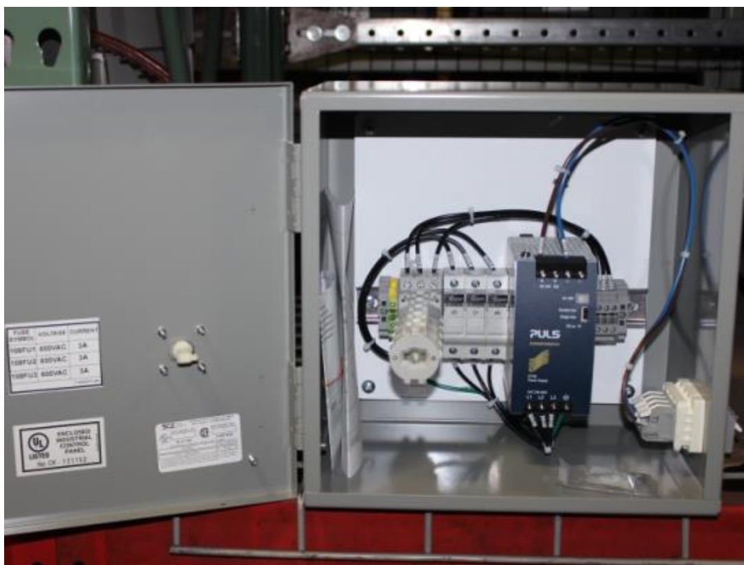
Motor Control Power Supply with Branch Circuit Protection (10A 480 VAC shown)
