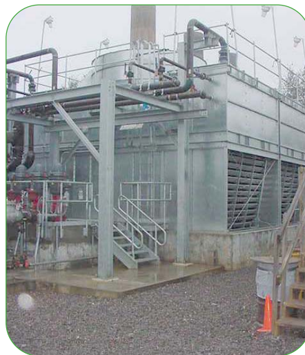
Installation on a concrete basin
