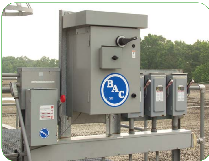
VFD & safety switch
