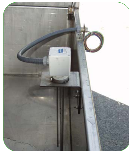
Electric water level control package
