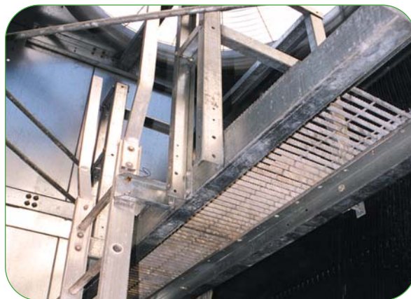
Internal ladder and service platform
