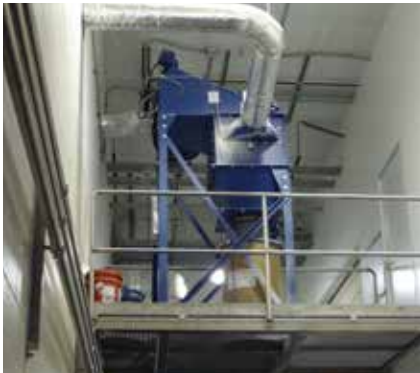
CPC on Milk Powder 1,200 cfm (2,038 m³/h)
