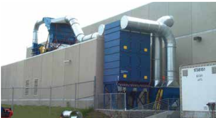
DLMC on Paper Dust 27,000 cfm (45,864 m³/h)
