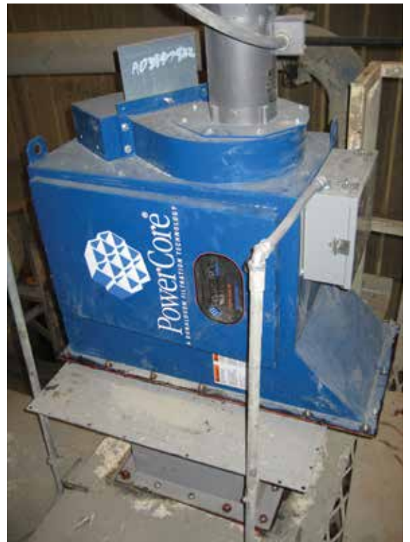
CPV - Feed Hopper 350 cfm (595 m 3 /h)
