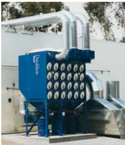
DFO on Metal Grinding 31,000 cfm (52,658 m 3 /h)
