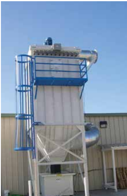
FS on Woodworking 20,000 cfm (33,973 m 3 /h)
