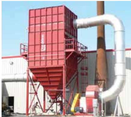
MB on Glass Processing 25,000 cfm (42,466 m³/h)
