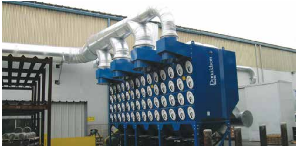
DFO on Grinding 74,000 cfm (125,700 m 3 /h)
