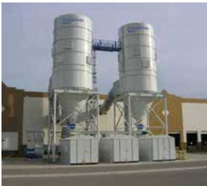
LP on Wood Dust 160,000 cfm (271,784 m 3 /h)
