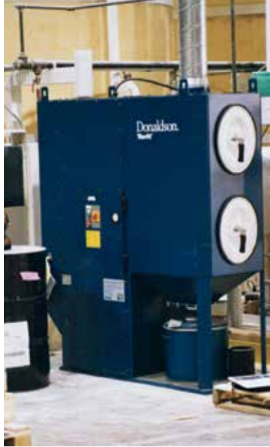
DFO on Paint & Pigment 1,200 cfm (2,038 m³/h)
