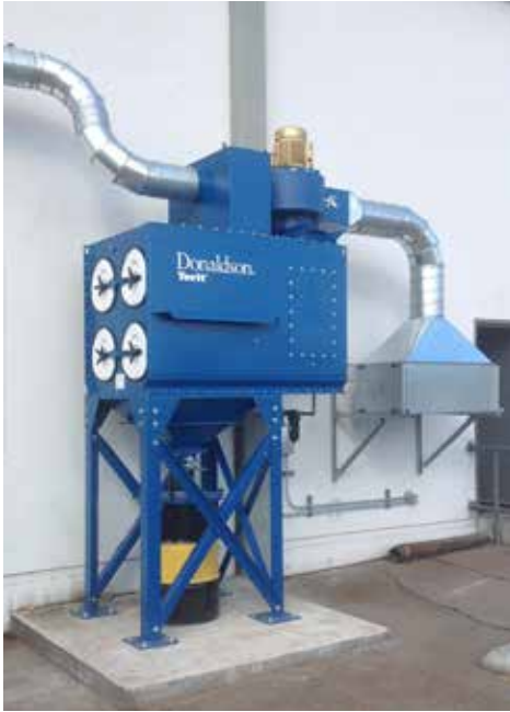
DFE on Rubber Hose Cutting 2,800 cfm (4,757 m³/h)
