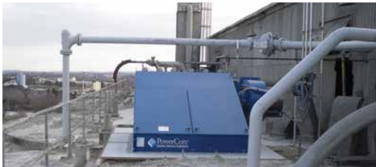
CPV - Multiple Cement Silos 4,800 cfm (8,154 m 3 /h)
