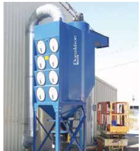
DFO on Plasma Cutting 5,000 cfm (8,493 m 3 /h)
