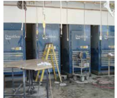
DWS on Granite Finishing 22,000 cfm (37,370 m³/h)
