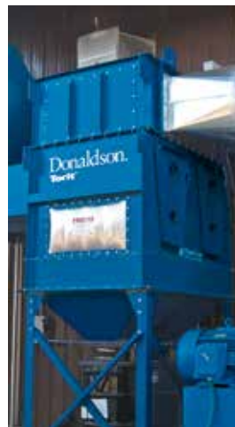
VH on Blasting 14,000 cfm (23,781 m 3 /h)
